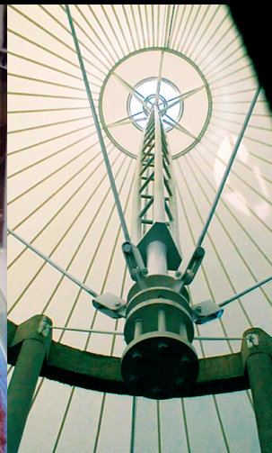
Fig. 2.29 Jacked flying mast
